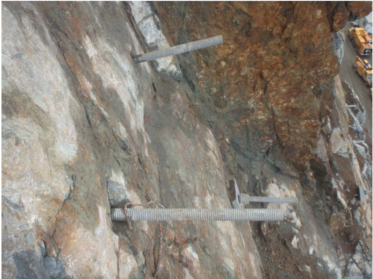
Figure 1. Anchors with no plates or grout on Cut 9, Segment 1. These anchors are to be tensioned rock bolts.
