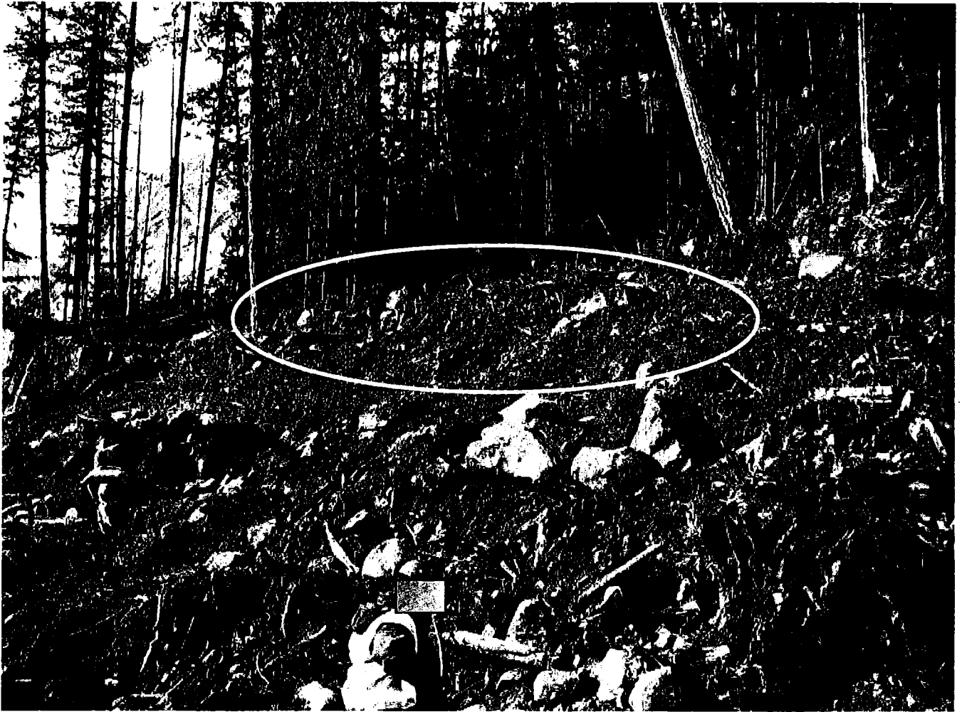
Figure 7. Rough area adjacent to previously machine-scaled ground.
