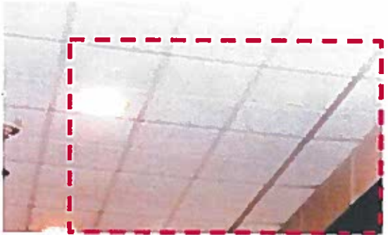
Fig. 87: A Water spot above this ceiling tile has not yet penetrated down.
