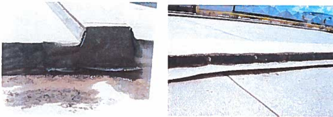
Fig. 55: Folded roofing membrane at this junction is difficult to seal.
