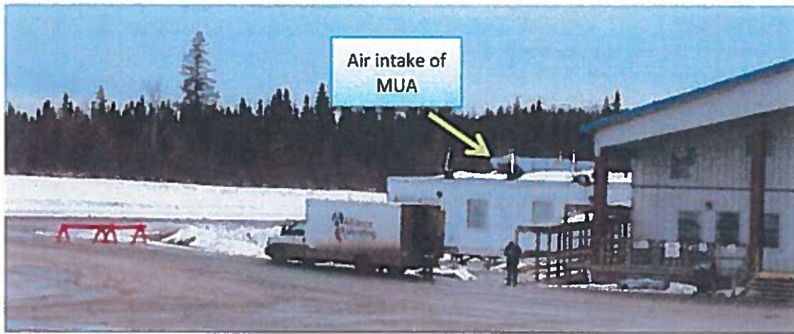
Fig. 152: Delivery truck idling near air intake of MUA
