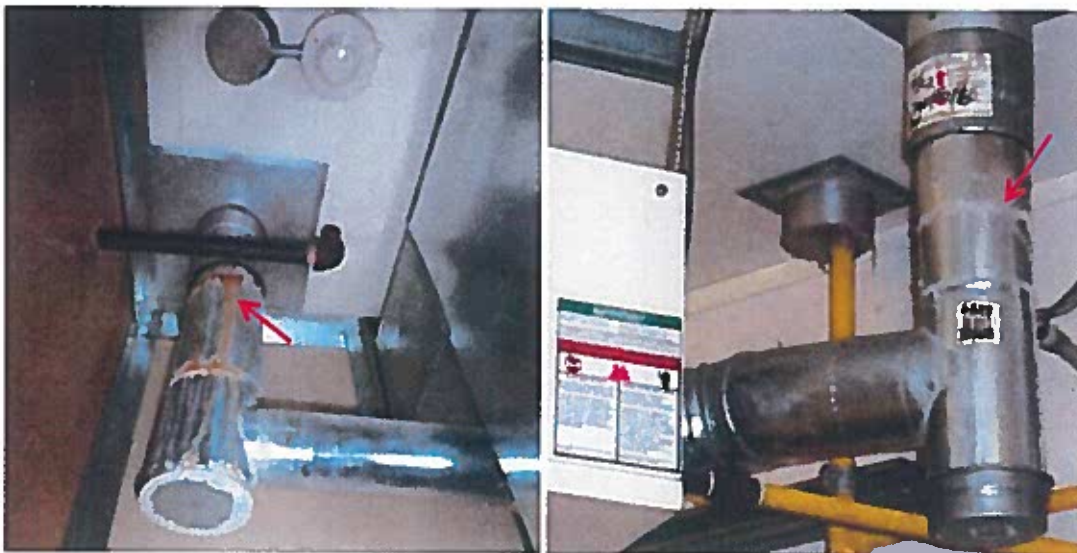
Fig. 124: Water leaking down the chimney of this furnace.
