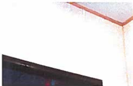
Fig. 83: Water streaks on the wall are evidence of past water leaks.
