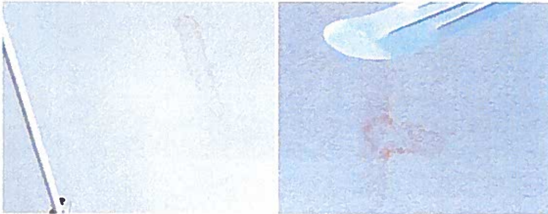
Figs. 96 & 97: Water staining on the sloped ceiling of the main lobby.
