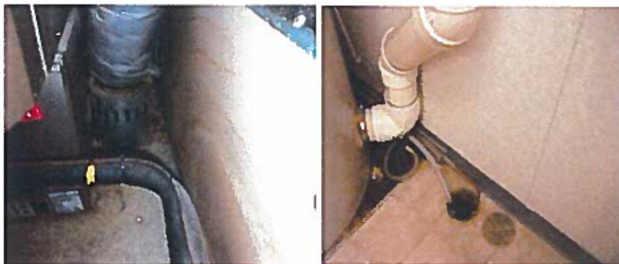
Fig. 139: Combustion air discharged onto the floor of the furnace room.
