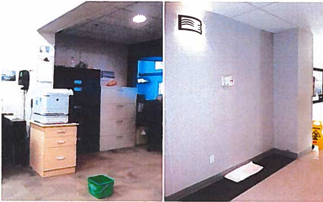
Fig. 76: Bucket collects water dripping from a module junction beam in the front office.
