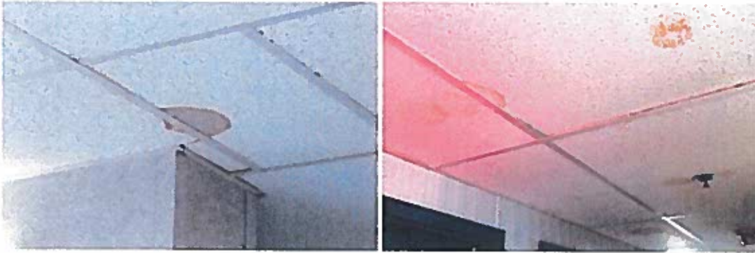
Figs. 65 & 66: Water staining on the ceiling of the corridors.
