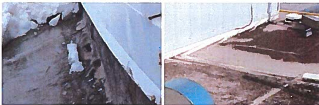
Fig. 63: Possible faults in the water-proof roofing membrane. Fig. 64: Soil accumulation is the result of water ponding on the roof.
