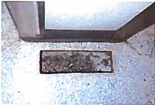
Fig. 143: Very dirty ducting inside the floor register.
