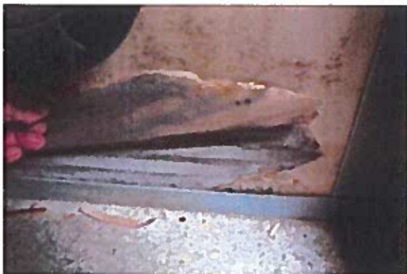
Fig. 128: Mould grows on the drywall close to the floor.
