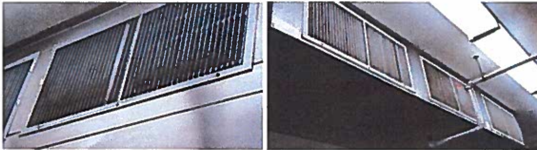
Figs. 104 and 105: Dirty air supply grilles in the Kitchen.
