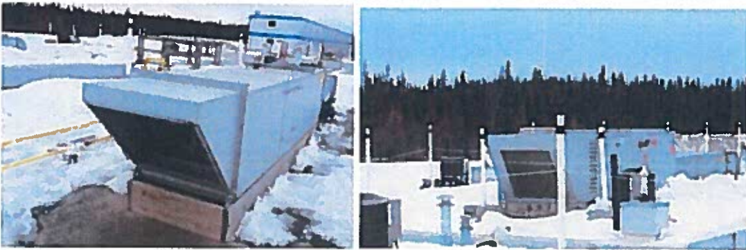
Fig. 147: Make-up air (MUA) unit for tempering the air intake
