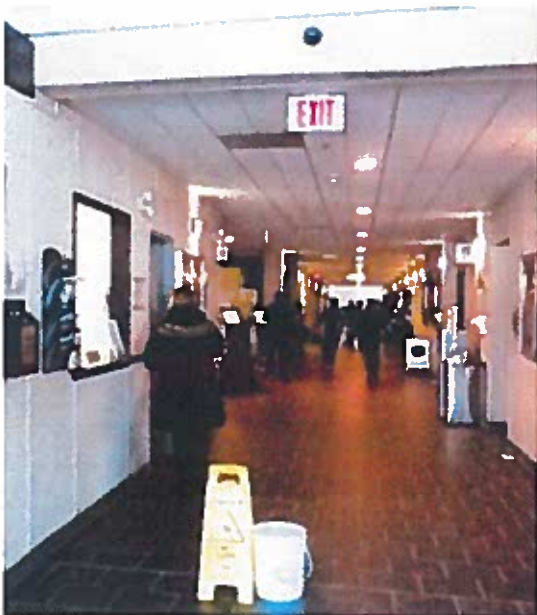
Fig. 74: Dripping water in the main corridor requires a bucket and caution sign.
