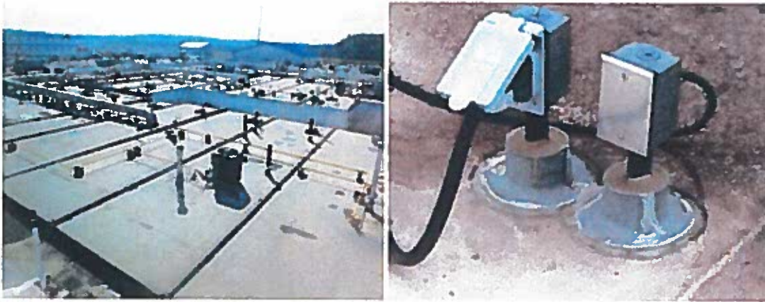
Fig. 57: There are many penetrations through the waterproofing membrane.
