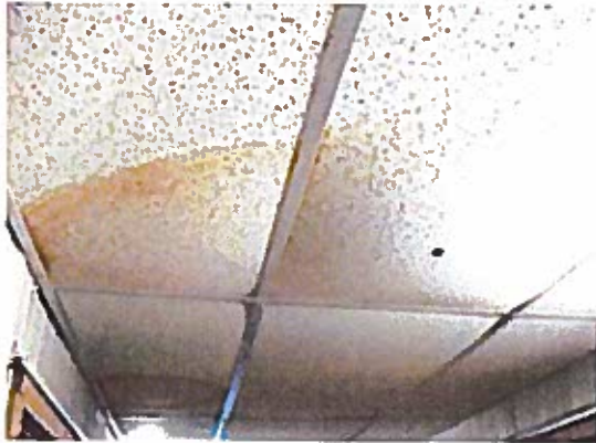
Fig. 69: Considerable water has leaked onto ceiling tiles in this residential corridor.
