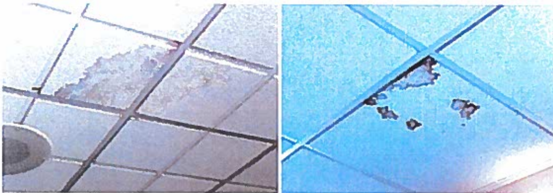
Figs. 70 & 71: Older water stains on the ceiling.
