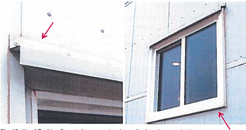
Fig. 42: Head flashing for windows are simply caulked to the metal siding.
