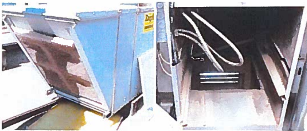
Fig. 154: Large amount of dust in the ambient air clogs up the air filters on the rooftop units.
