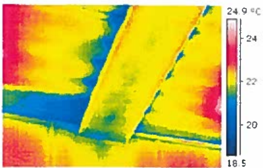
Fig. 86: Cold signatures in the ceiling of the Pakhismtakh (conference room).
