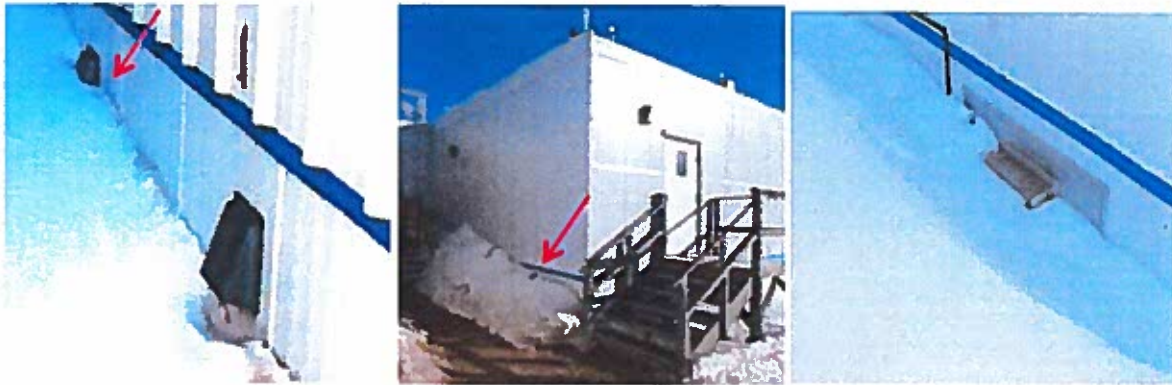
Fig. 136: The air intake hood at the back of photo is blocked with snow.
