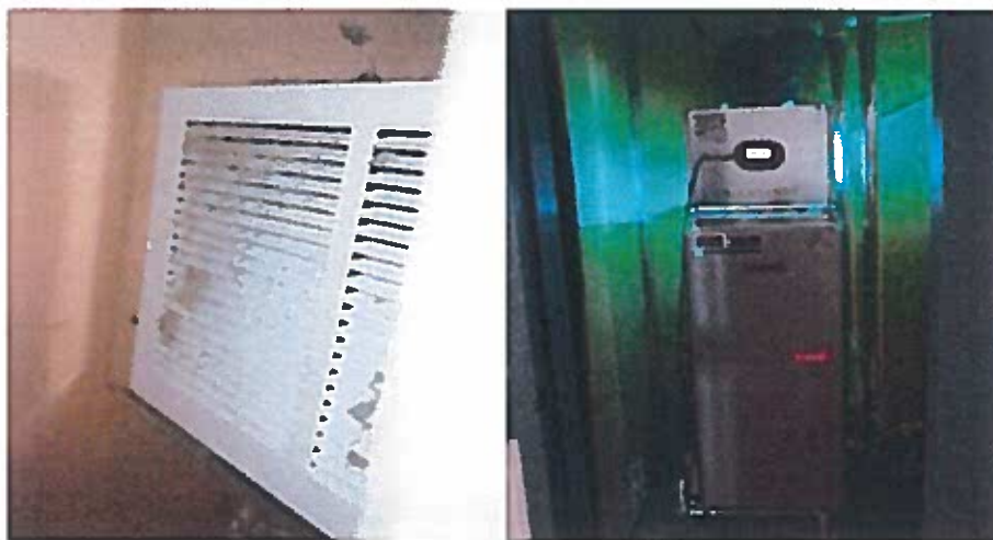
Fig. 129: Dust and hair on the return air grill on the furnace.
