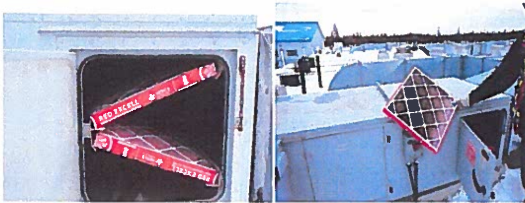
Fig. 149: Typical placement of the panel filters in a make-up air unit
