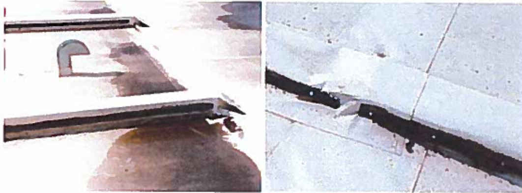
Fig. 53: Junctions between units are difficult to seal properly.
