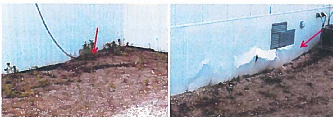
Figs. 17 & 18: Gaps in the foundation skirt allow animals to enter the crawl space.
