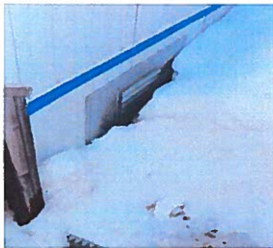
Fig. 33: This air intake grille is partly covered with snow.
