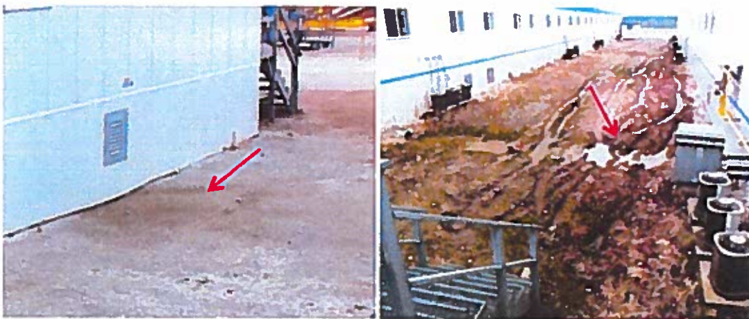
Fig. 13: Evidence of surface water runoff into the crawl space.
