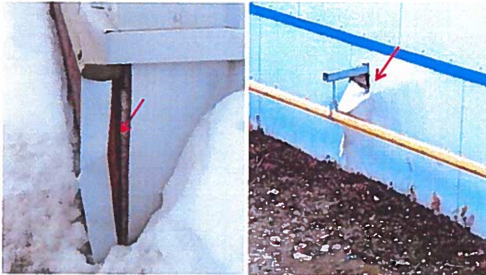
Fig. 40: This damaged corner exposes the wood to weathering.
