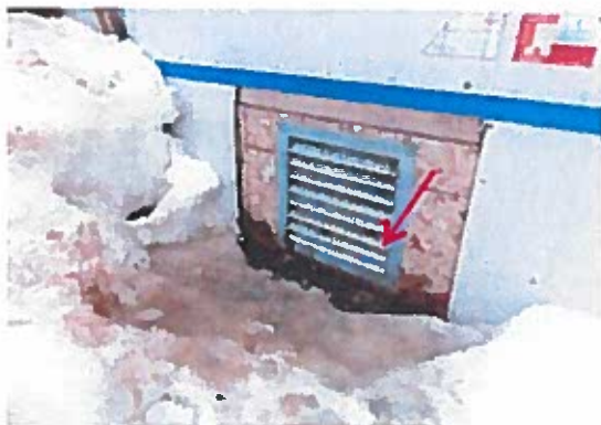
Fig. 36: Exposed OSB wood for the skirting will rot and is not an effective barrier to rodents.
