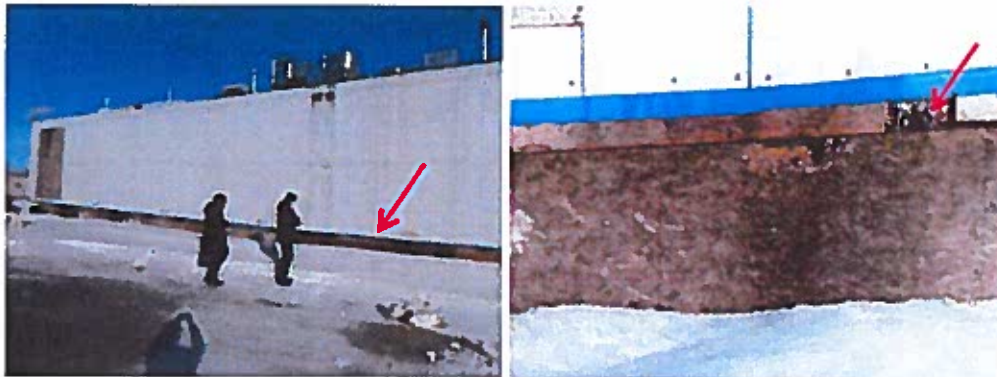
Fig. 37: Entire length of this skirting around the kitchen has exposed untreated OSB wood.
