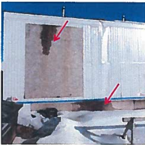
Fig. 39: This OSB is wet and water damaged, allowing water to seep into the wall assembly.
