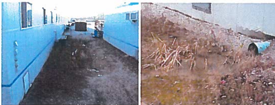
Fig. 15: Water accumulation near the building is a long-term problem as indicated by these cattails growing in a pond between wings at Wapasu Creek East.
