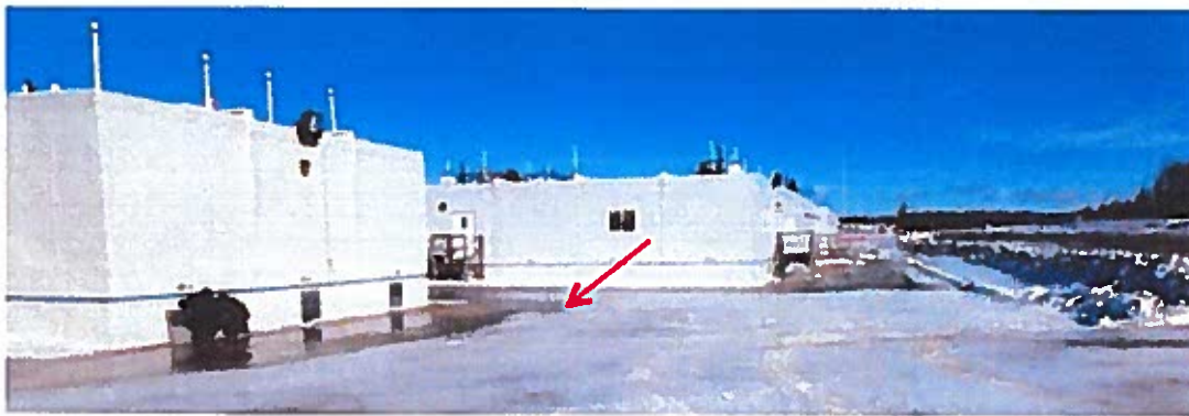
Fig. 19: Surface drainage flows toward the building causes flooding the crawl space. Location: Wapasu Creek West.
