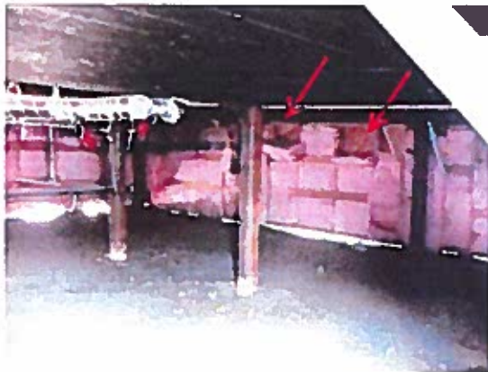
Fig. 29: Insulation falling off the crawl space walls.
