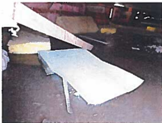
Fig. 22: Debris including insulation and wood are left inside this crawl space.
