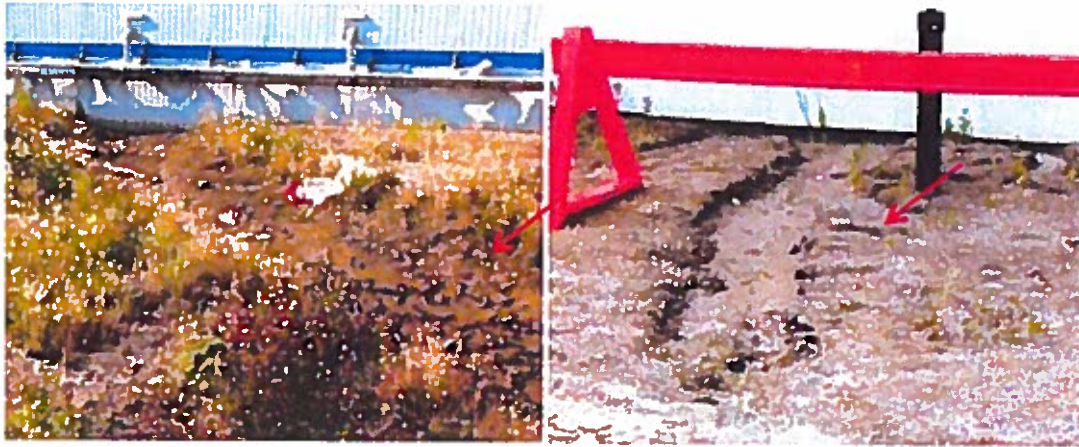
Figs. 11 & 12: Water migrating into the crawl space causes this ground erosion. Location: Henday.
