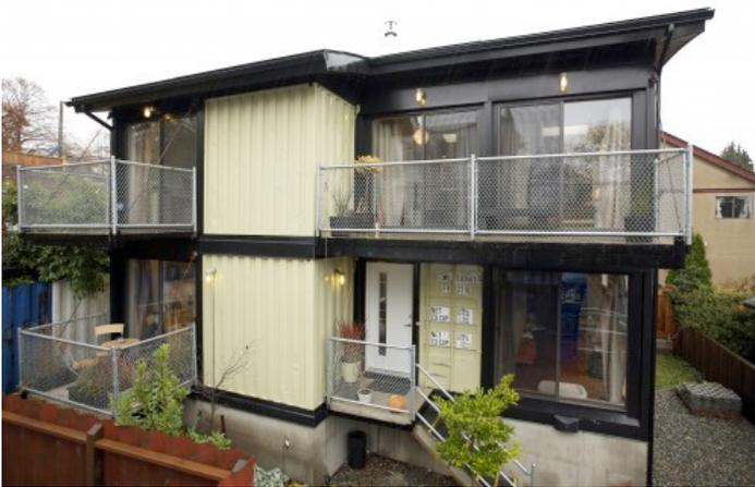
*TO LEFT: Zigloo Domestique is a custom home in Victoria, B.C. Architect Keith Dewey reused eight 20-foot-long shipping containers to create its frame. Open floor plans such as this can cost less to build using shipping containers than wood or concrete, because long steel beams are included in the price of the used container. Photo courtesy of Keith Dewey*
