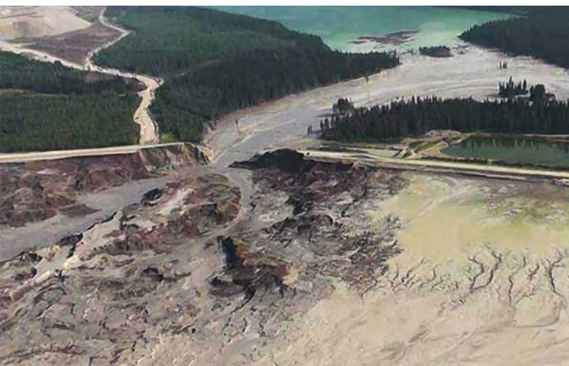
The aftermath of a tailings pond failure at Mount Polley mine, 2014. Photo: Cariboo Regional District.
