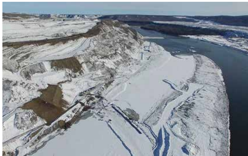
Site C under construction, March 2017. Photo by Zoë Ducklow.
