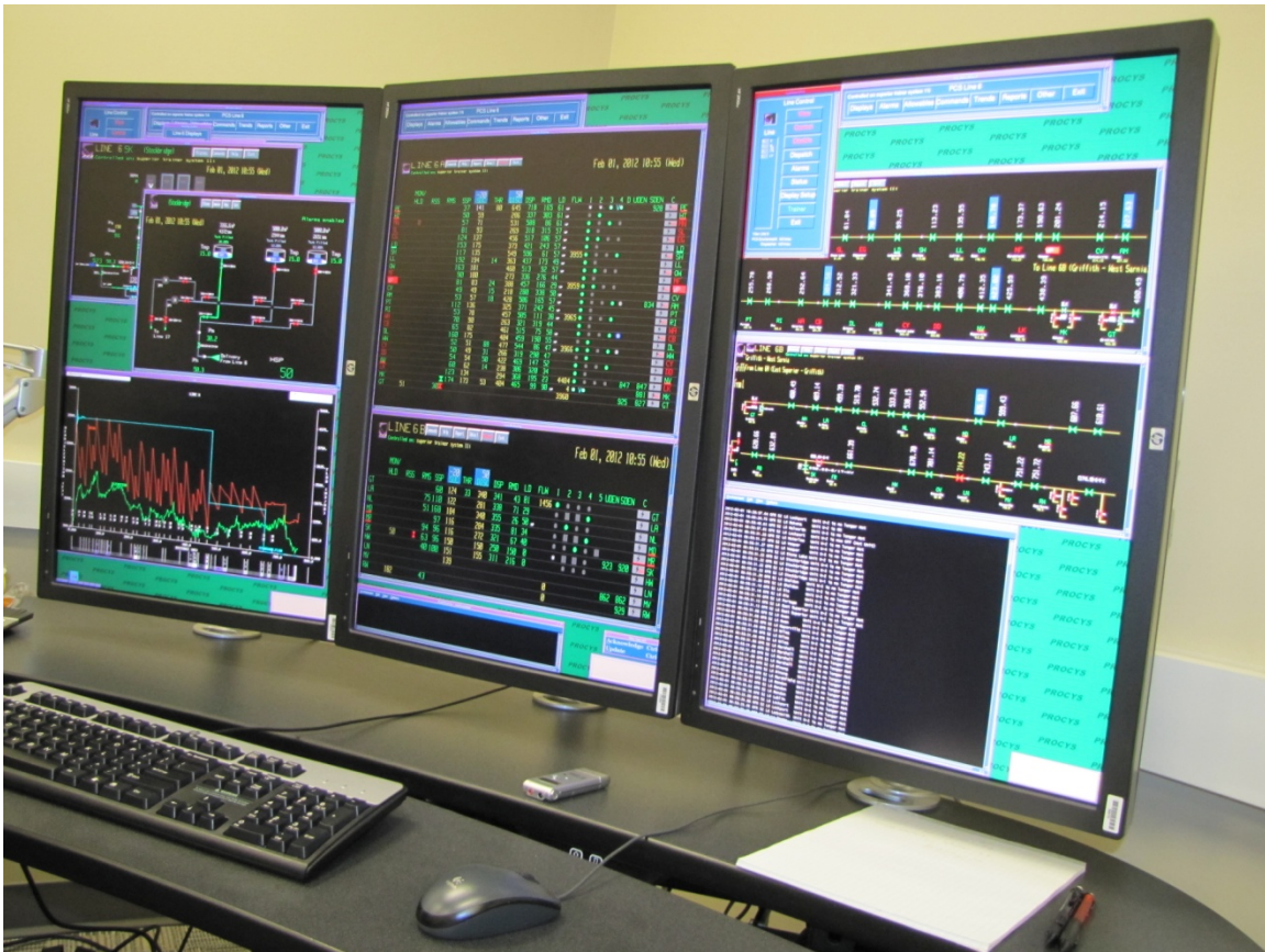
Figure 2: Simulated Training Console; operations SCADA screens displaying simulated Line 6A & 6B on February 1, 2012, Source: NTSB. See Appendix 2
