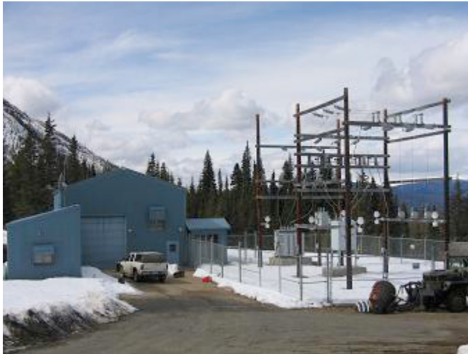
Photo: Power house for the Hluey Lake hydro project. The Hluey Lake hydro project, with a peak power capacity of 3 MW, currently provides year-round electricity to the community of Dease Lake. A second turbine could be added to expand its capacity to 6 MW.
